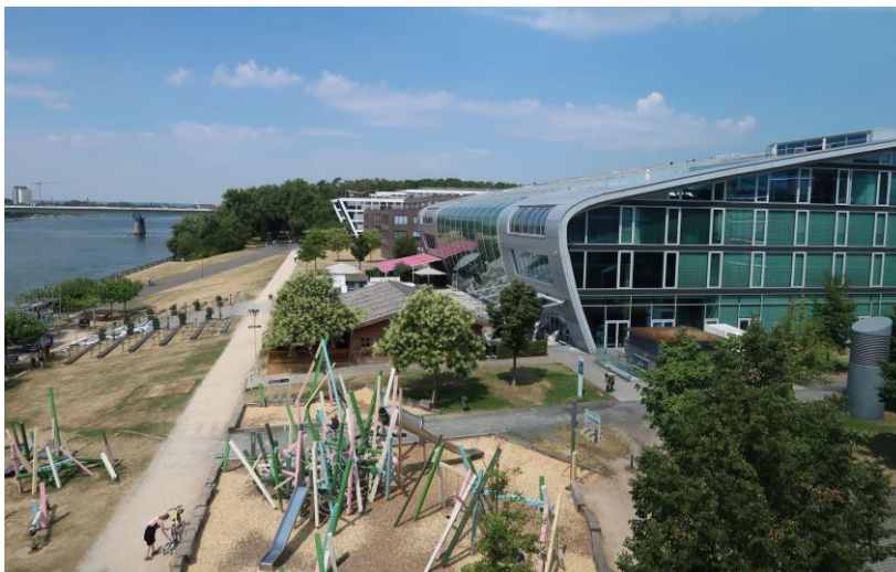
Supply of cold in the summer and heat in the winter: A hotel and two office buildings in Bonn use an underground aquifer for this purpose. (Photo: Paul Fleuchaus, KIT)
