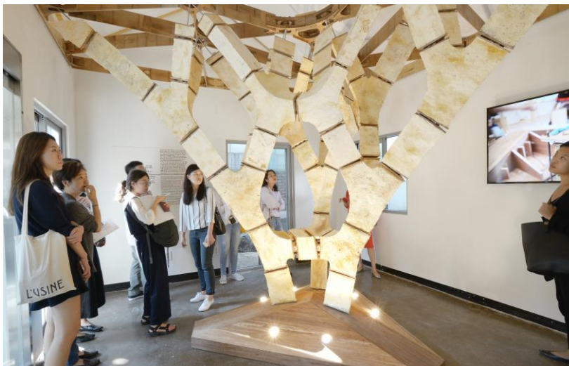
The “Mycotree,” a structure of fungal mycelium and bamboo. The geometry was optimized and made load-bearing using 3D graphic statics methods. (Photo: Carlina Terteris)
