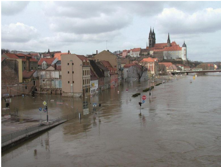
Flood in Meißen in 2006: Due to the rapid increase in the water level, time for early warning is short. (Photo: GFZ, German Research Centre for Geosciences)
