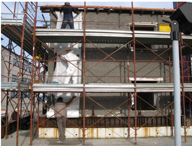
KIT researchers tested the protective effect of the seismic wallpaper on a two—storied building in the Italian city of Pavia. (Photo: Moritz Urban)
