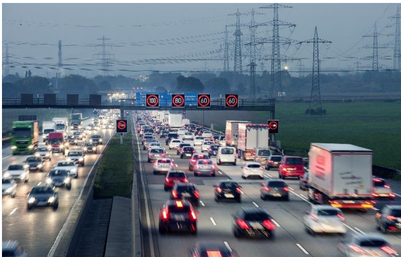
Traffic management systems enhance traffic safety on freeways. Here, the morning rush hour at the Frankfurt northwest interchange is shown. (Photo: Hessen Mobil Straßen- und Verkehrsmanagement)
