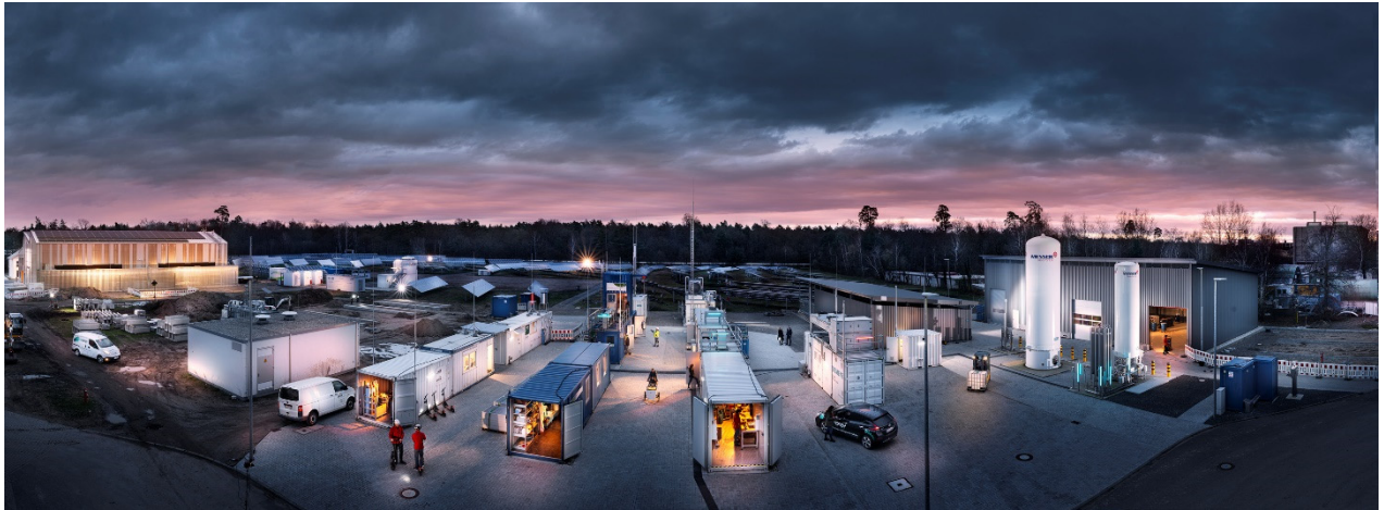
Energy Lab 2.0 on the campus of KIT is Europe's largest research infrastructure for renewable energy. Here, studies focus on the smart interconnection of environmentally friendly energy producers and storage methods, among others. (Photo: Markus Breig and Amadeus Bramsiepe, KIT)
