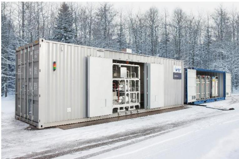
The compact pilot plant used in the SOLETAIR project is designed for decentralized production, fits into a shipping container, and can be extended modularly. (Photo: VTT)
