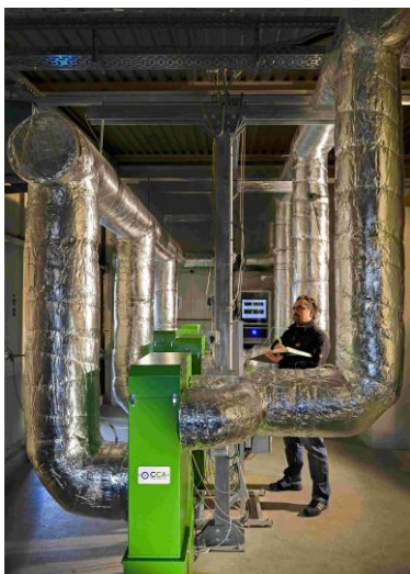
The CCA separator (light green) efficiently removes fine dust from flue gas of wood-fired boiler systems. (Photo: KIT)
