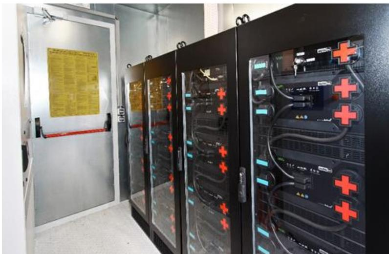
*The batteries store solar power and feed it into the mains of HIU, if required. (Photo: Frederik Elschenbroich, ads-tec)*
