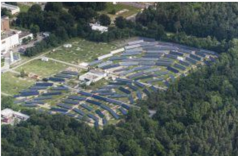
Thanks to modern battery and information technologies, solar power produced by the KIT solar power storage park is reliably fed into the grid. (Photo: Markus Breig, KIT)
