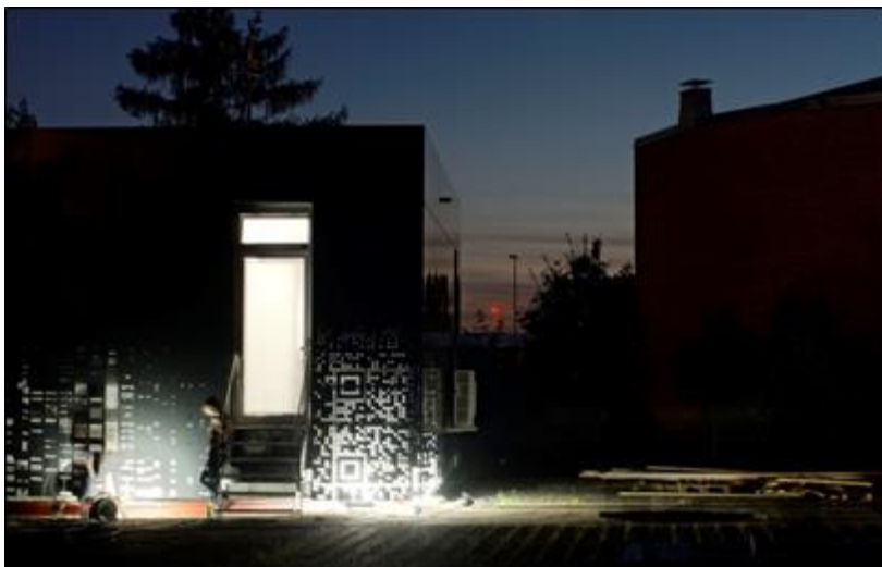
LOBSTER at night: The front is made of aluminum composite boards milled in a computer-supported manner. (Photo: Robin Nagel/Moritz Karl)
