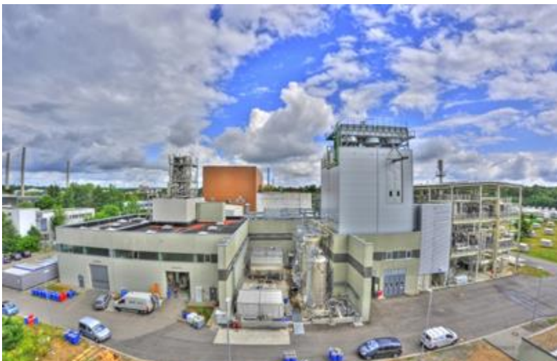
The bioliq ® plant at KIT: In a multi-stage process, high-quality synthetic fuels are produced from straw and other biogenous residues. (Photo: KIT/Tom Zevaco)
