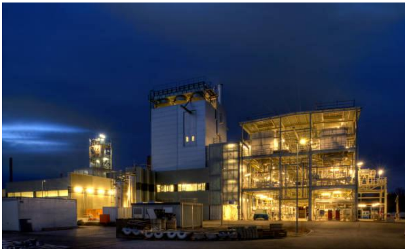
The bioliq ® plant at the KIT: in a multi-stage process, high-grade synthetic fuels are produced from straw and other biogenic residues. (photo: Markus Breig)
