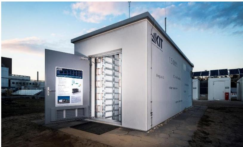
*Highly reliable and efficient: The new lithium-ion battery storage system in test run at Energy Lab 2.0 can be used as district storage system for local grid stabilization. (Photo: Amadeus Bramsiepe, KIT)*
