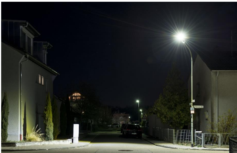
The new street lights tested in Maxdorf consume less power and are much brighter. (Photo: Tanja Meißner/KIT)
