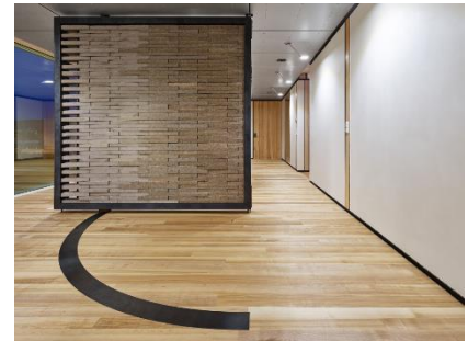
Mineral waste materials were turned into new bricks which were then used without mortar in order to ensure later sorting and separation of materials. (Photo: Zoëy Braun)
