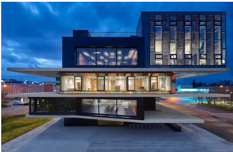
The residential unit is made of primary resources, such as untreated silver fir wood, newly developed construction materials, and recycled resources. (Photo: Zooey Braun)
