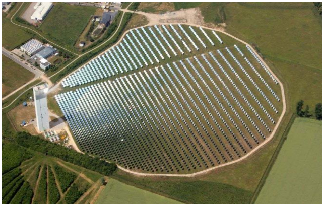
The sulfur-based technology for the storage of solar energy will be tested at the Jülich solar power tower. (Photo: DLR)
