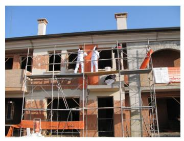
Walls are "papered" with long lengths of seismic fabric and then plastered. In case of emergency, the seismic fabric holds the debris and keeps escape routes free from obstruction. (Photo: M. Urban/KIT)
